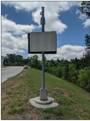
F6. Rear Sign Pole with Camera/Detection & Antenna (Front/Rear)
