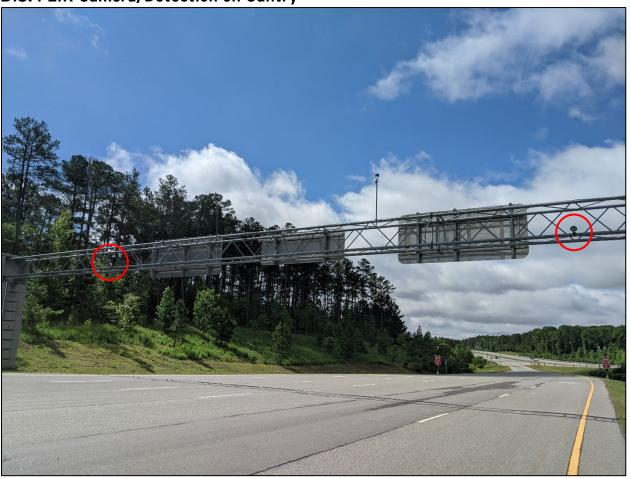
B14. FLIR Camera/Detection on Gantry (Front/Rear)
